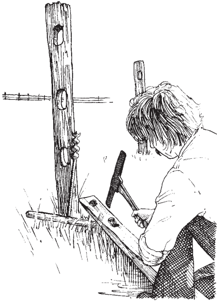
Chop holes through fence posts with a narrow-bitted mortising axe.
