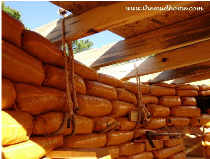
Joists tied down with ropes. (My roof ain't going nowhere ).
