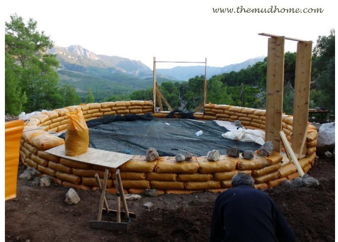
Earth-filled sack on the runner.
