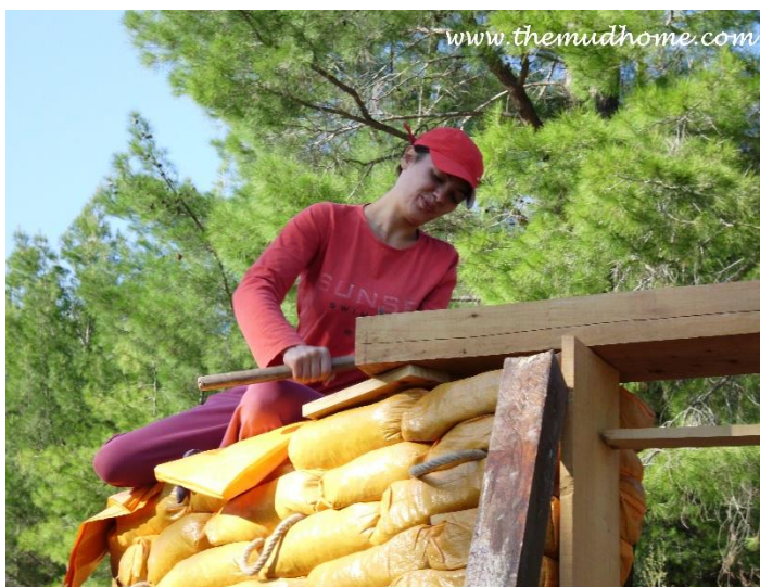
Esra banging in an anchor to stop the lintel sliding.
