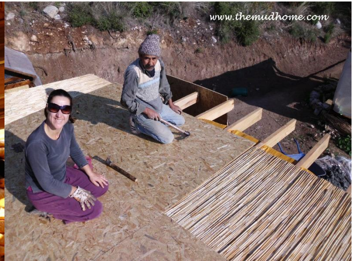
Bamboo matting under the OSB.
