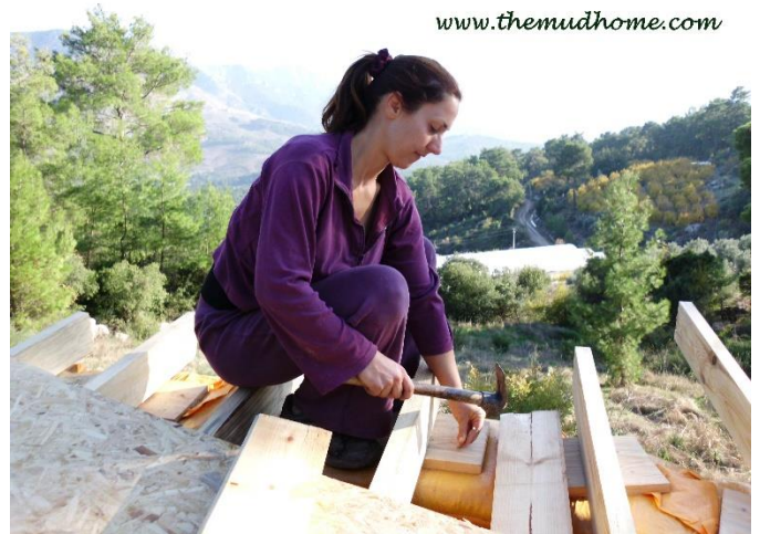
Each rafter was anchored using wooden slats.
