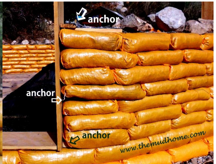
Three anchors here
