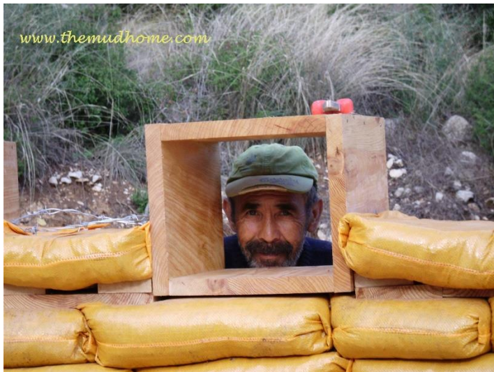
Bag butts rammed against frame, atop two anchors.
