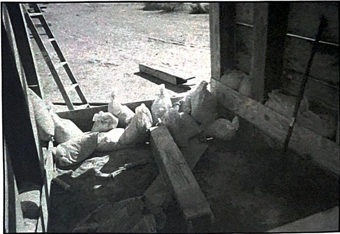
The sleeping cube. Sandbags fill the voids and are sheathed with scrap plywood. The posts, after being anchored with cement and rebar, are filled with dirt and gravel.
