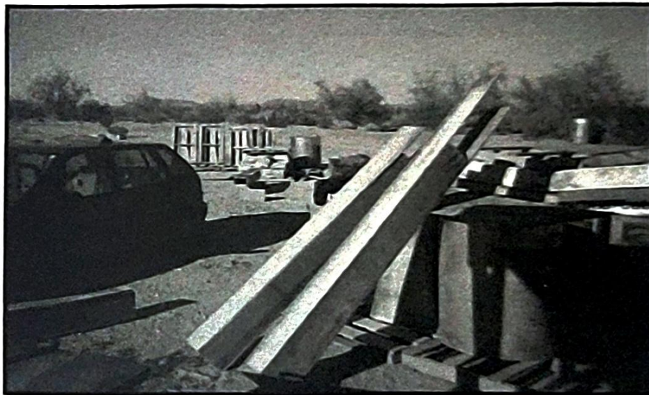
Glue-nailing together the posts and beams.
