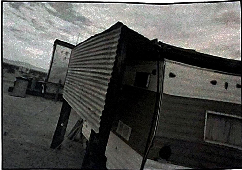
Sheet metal awnings for sun and wind protection.
