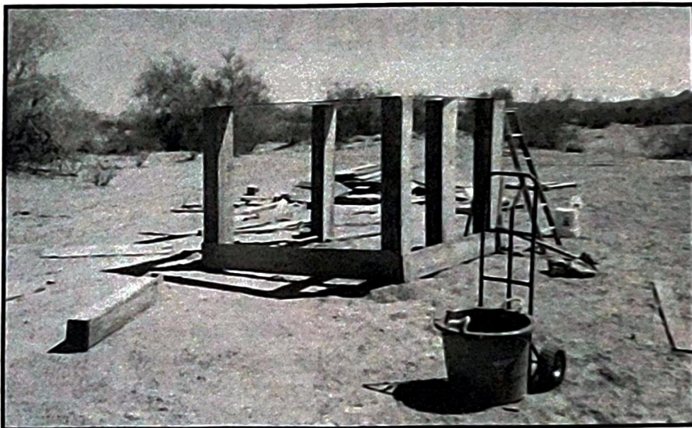
The beginning of the sleeping cube. Hollow posts are used in lieu of studs.
