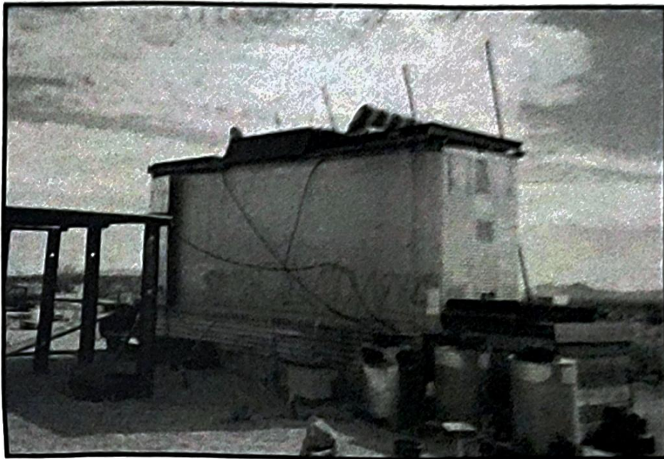
The Hobo collects the runoff from the infrequent desert cloudbursts. The water runs from roof gutters through tubing and is collected in tanks.
