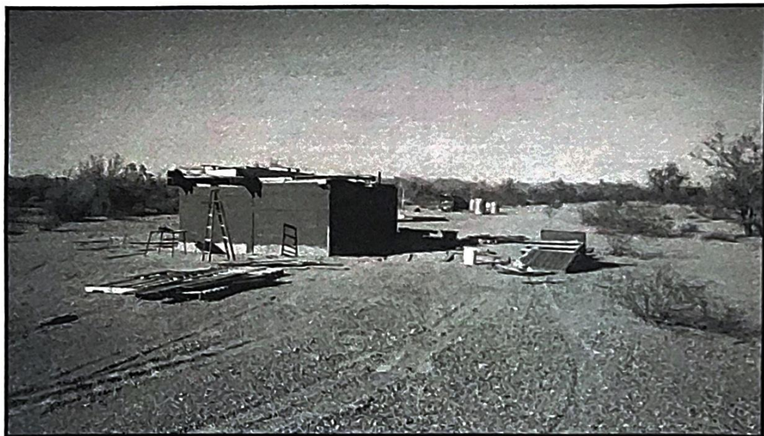
Overview of the hogan. The roof is held down with pallets and tires.
