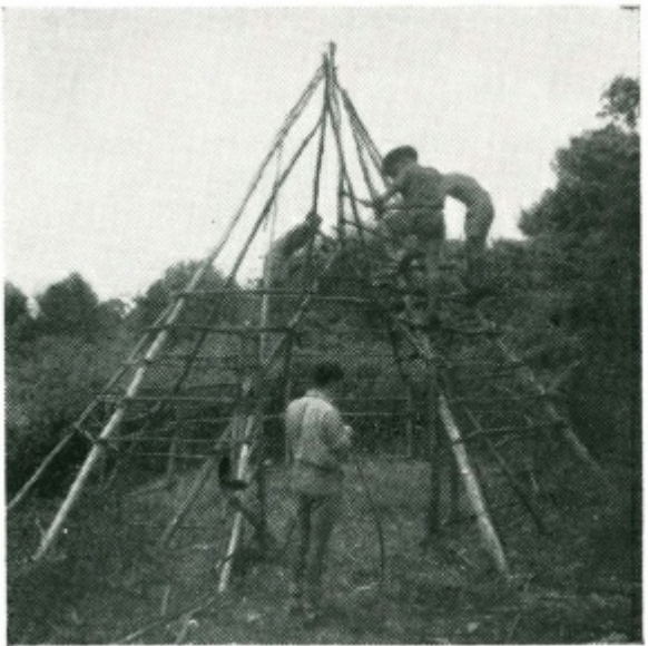
(4) One and a half hours after start: Thatching battens are nearly all lashed on, door is complete, ready for thatching.
