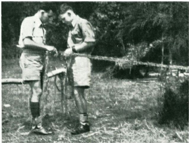
Joining the strands prior to lay up.
