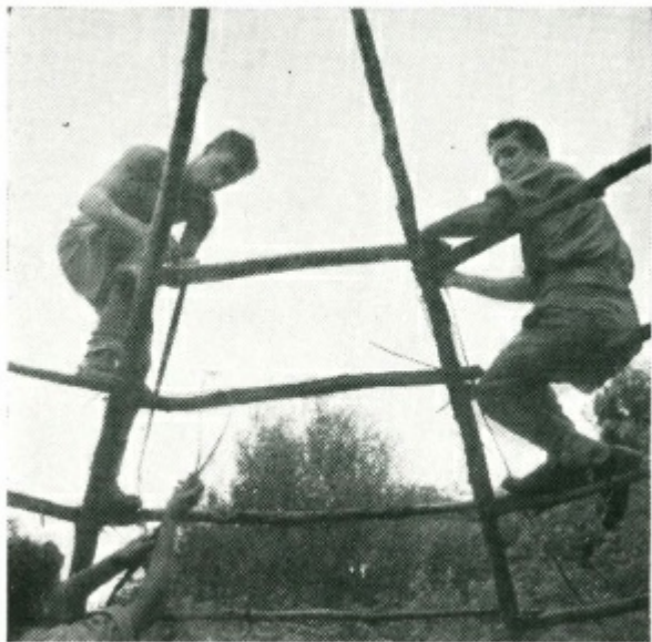
(3) Lashing on the thatching — battens to the rafters. Note how the lower battens must be strong enough to bear a man's weight.
