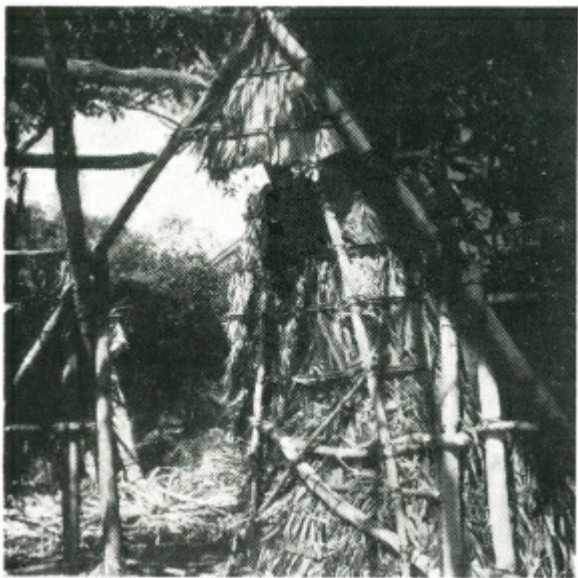
(5) Two and a half hours after start: The door is completely thatched, and the thatching is well under way on the roof.
